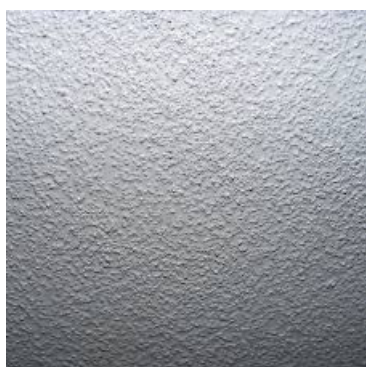
Figure 19: A rough grit-filled surface collects dirt up to 150 mm
