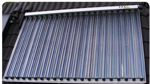
Evacuated tube solar collector installed on a roof. Source: RaBoe/Wikipedia/commons.wikimedia.org/wiki/File:Vakuu-roehren-kollektor_01.jpg
