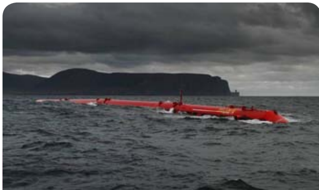
A Pelamis wave energy converter (linear absorber). Source: Wikimedia
