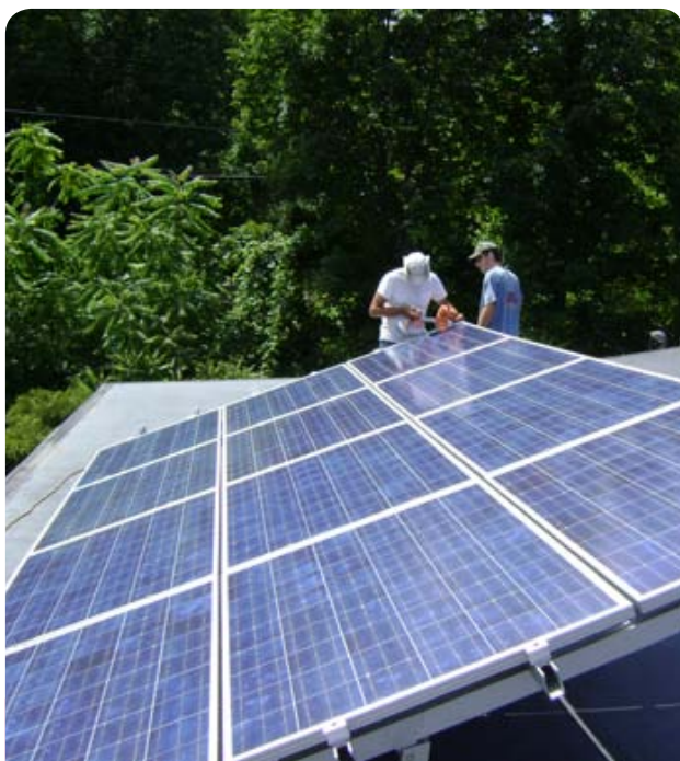
Two workers installing a tilt-up photovoltaic array on a roof. Source: Labraun90/Wikimedia
