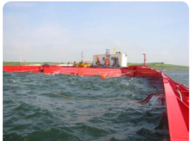
A Wave Dragon wave power facility. This is a example of an overtopping terminator. Source: Erik Friis-Madsen/Wikipedia
