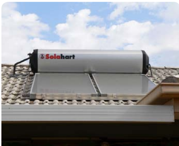
A Solarhart brand solar hot water panel and integrated tank on a house roof in Australia. Source: Fairv8, Wikimedia Commons
